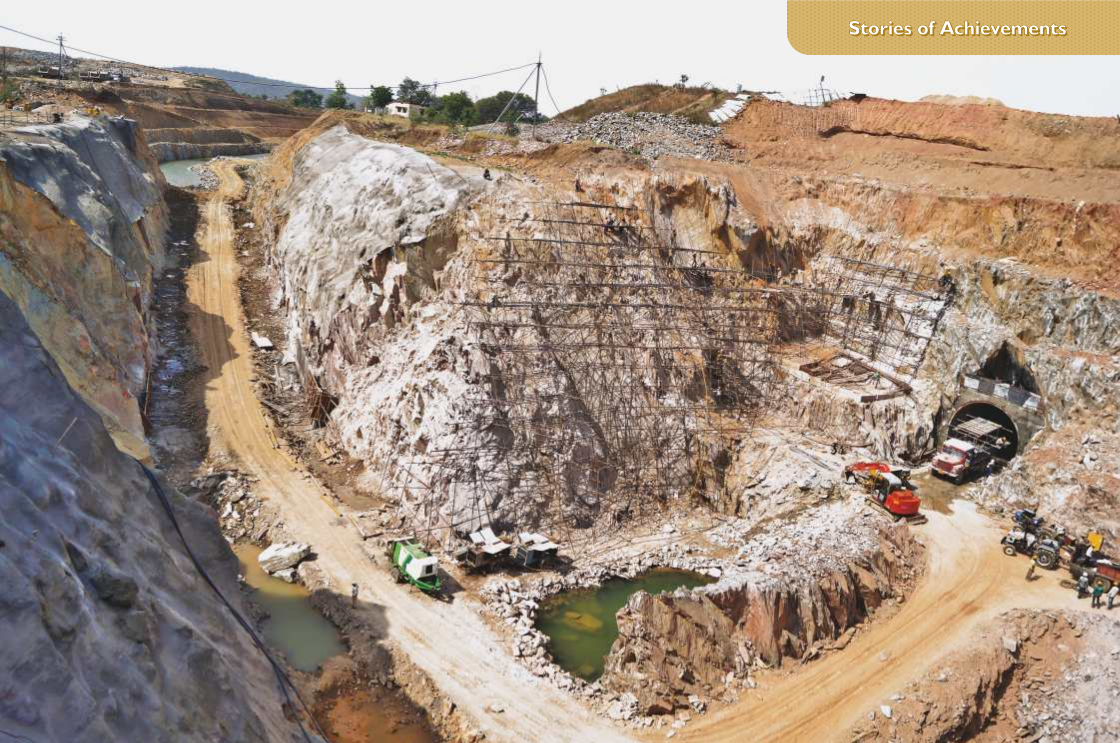
Biggest Hydro Power Project in Vidarbha
